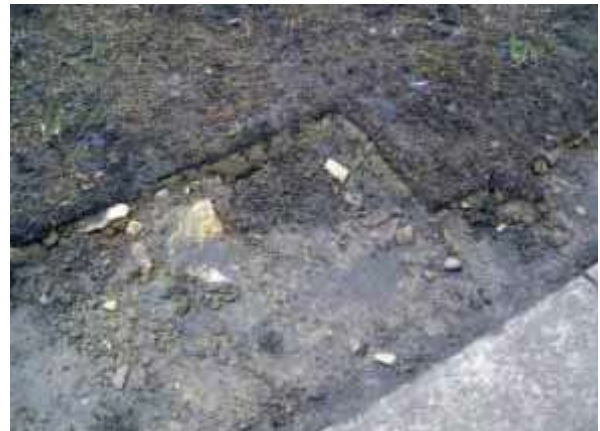
Surface water running onto adjacent paving
