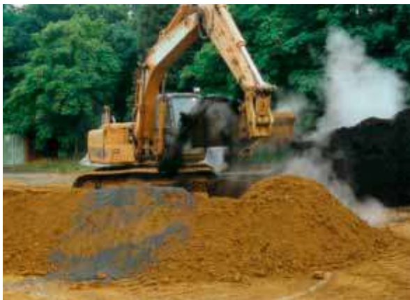
Blending organic matter with mineral material
