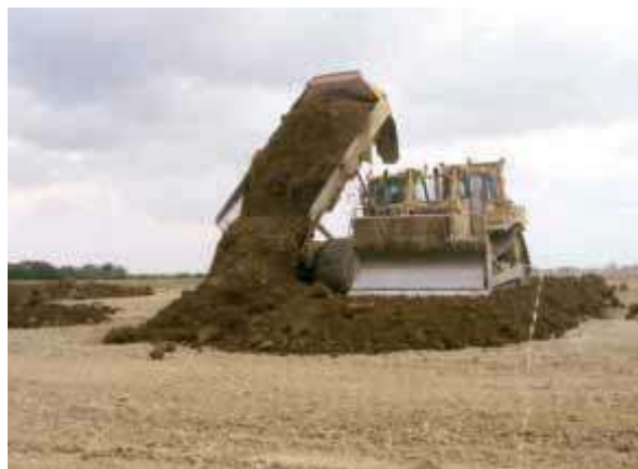
Starting a 'peninsula' of topsoil
