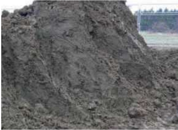
Topsoil stockpiled when wet and plastic
