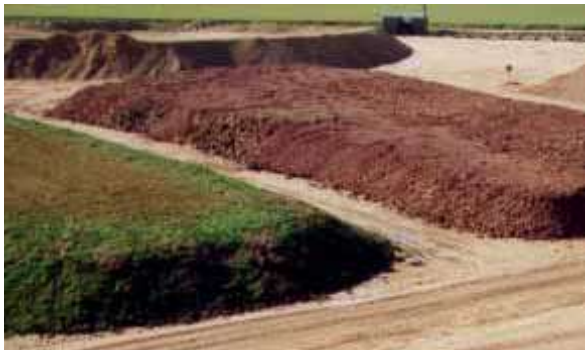
Clearly defined stockpiling of different soil materials
